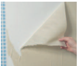
Wait 5-10 minutes and peel off backing
